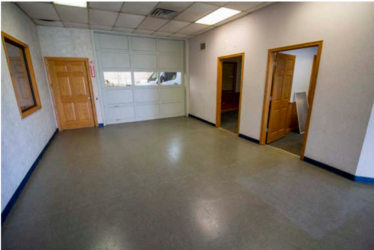
OVERHEAD DOOR TO WORKSHOP
